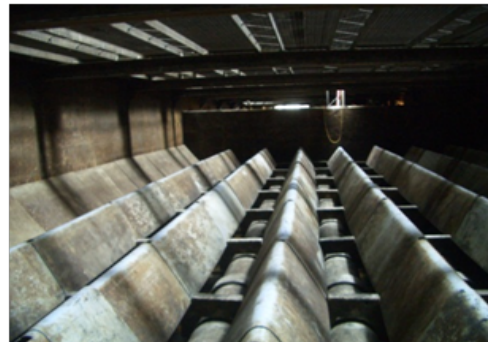
Baffle Plates in Sedimentation Pond
